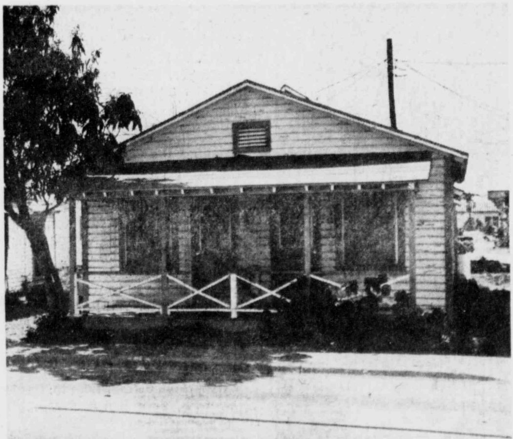
A Wooden Shack on Cement Blocks ... the tenant enjoys free water when it rains
